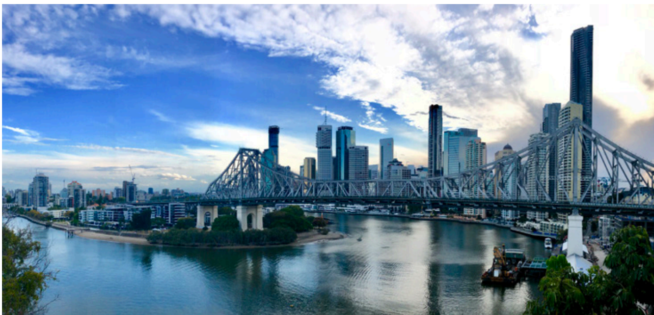
Story Bridge in Brisbane, Australia.
